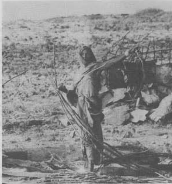
The skins (itile) and woven sisal mats (dasse) are first removed from the outside of the house, then the twines holding the house pole (utuba, dedee) joints together are untied; these are made of wild sisal (algi) or certain grasses.
