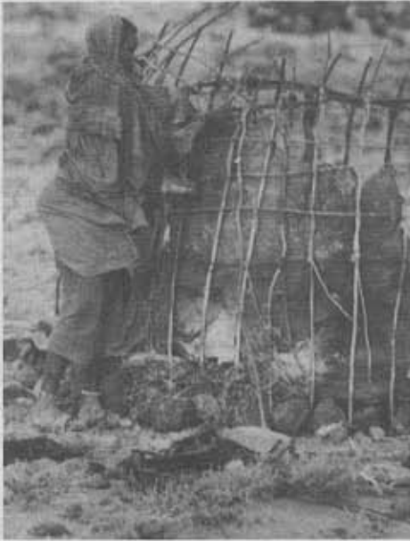
The house poles, made from strong but supple branches or saplings of Cordia gharaf/sinensis (madera) or Grewia bicolor/trichocarpa (aroessa), are tied together with ropes (haath algi) made from woven wild sisal fibers.
